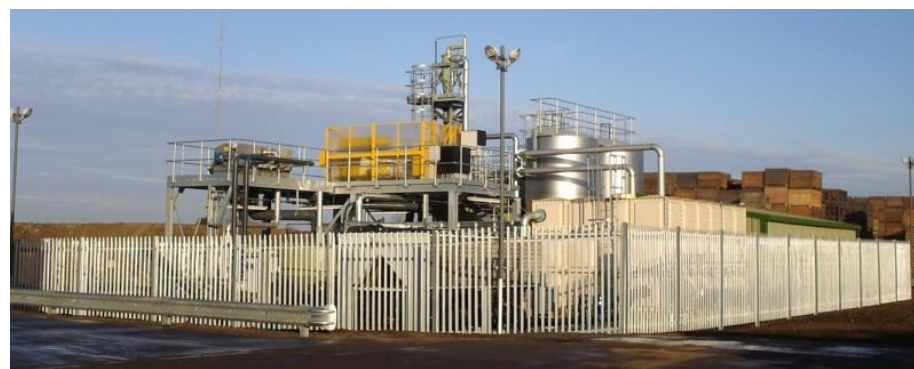
Greenvale's Cambridgeshire cascade washing plant (Source: Greenvale AP)
