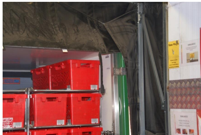
Seals around vehicle doors in the loading bay help to maintain strict temperature control Source: Oakdene Hollins
